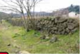
12 Stone Wall Along the River
