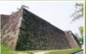
4 Main Compound North Stone Wall
