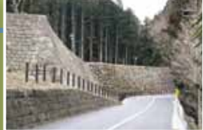
6 Main Compound Northwest Stone Wall
