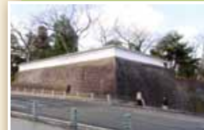
2 Otemon Gate North Earthen Wall (extant)
